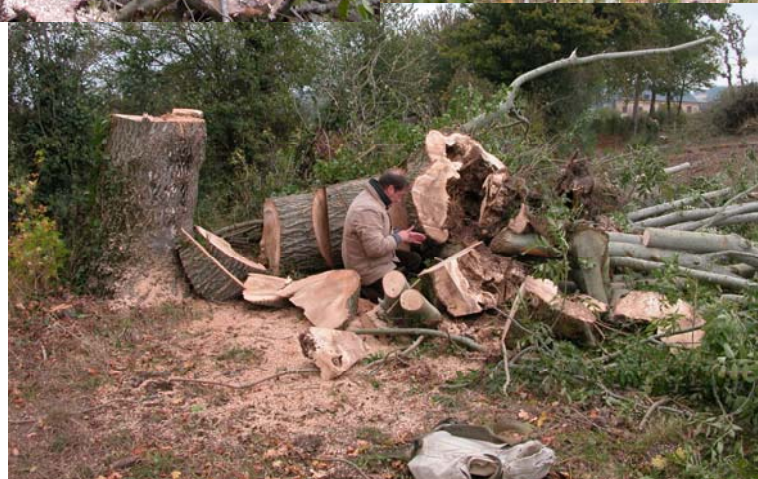
Trees felled as part of the motorway works are closely inspected for signs of Osmoderma
