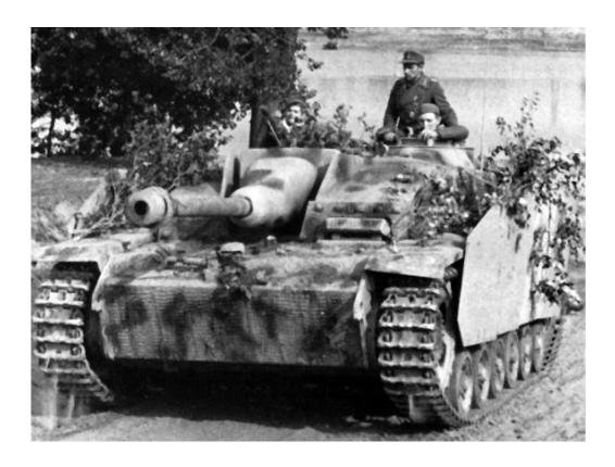
Many StuG's carried spare track links on the front walls of hulls and superstructures for added protection and therefore acting as extra armour.
